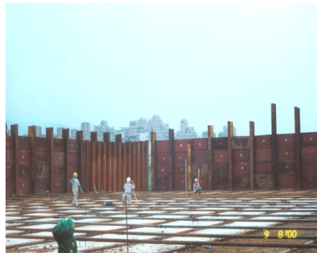
Figure 23 EPS level measurement
