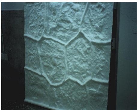
Figure 8 EPS special formwork
