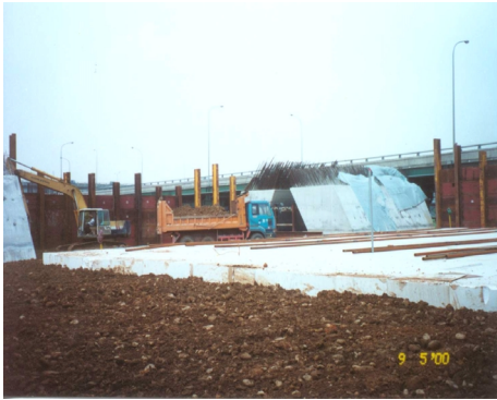
Figure 24 EPS backfill
